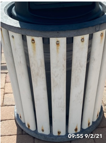
Observation 11 Remove rust stains from trash receptacles at Swim Club.
