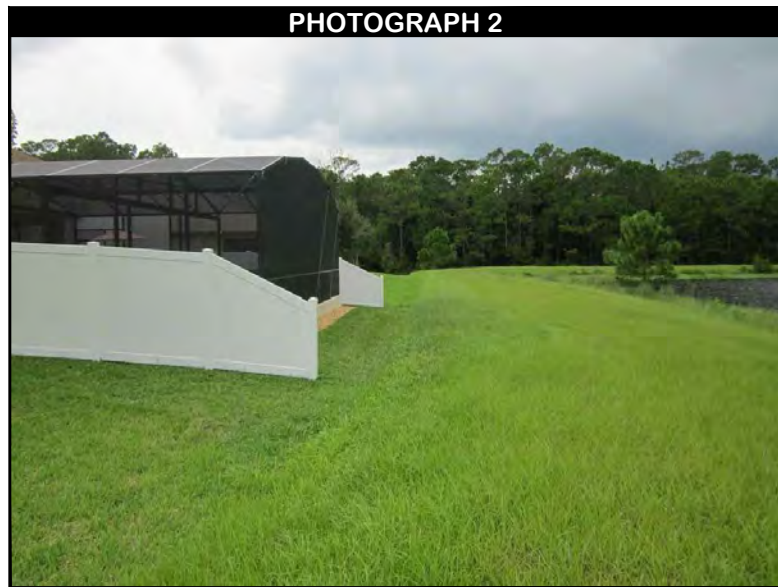
LOOKING WEST AT THE FENCE AND POOL DECK ENCROACHMENTS WITHIN THE REAR YARD SWALE BEHIND 3170 DARK SKY DRIVE.
