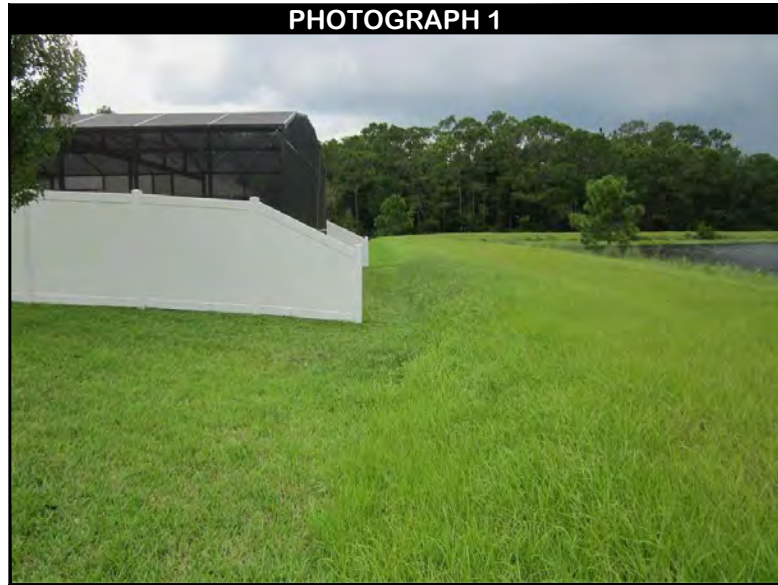
LOOKING WEST AT THE REAR YARD SWALE BETWEEN 3168 AND 3170 DARK SKY DRIVE.
