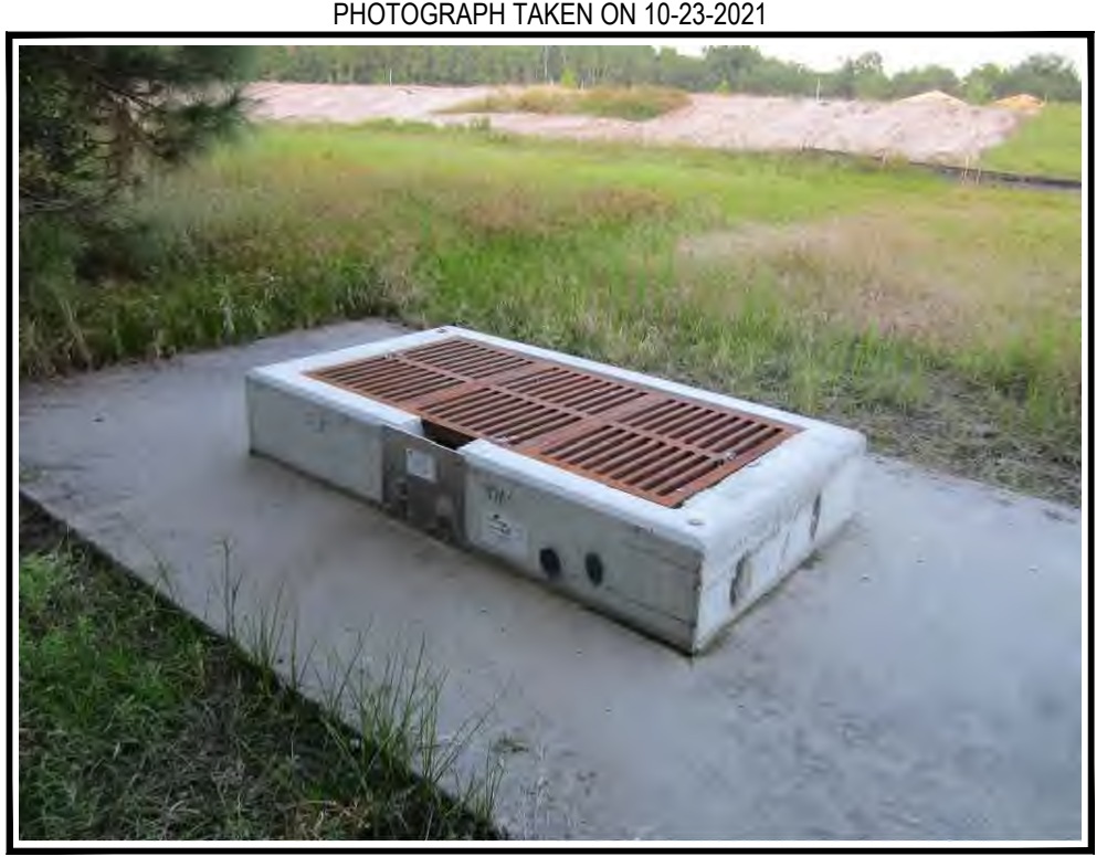
EXISTING OVERFLOW STRUCTURE, CONCRETE APRON AND CIRCULAR ORIFICES
