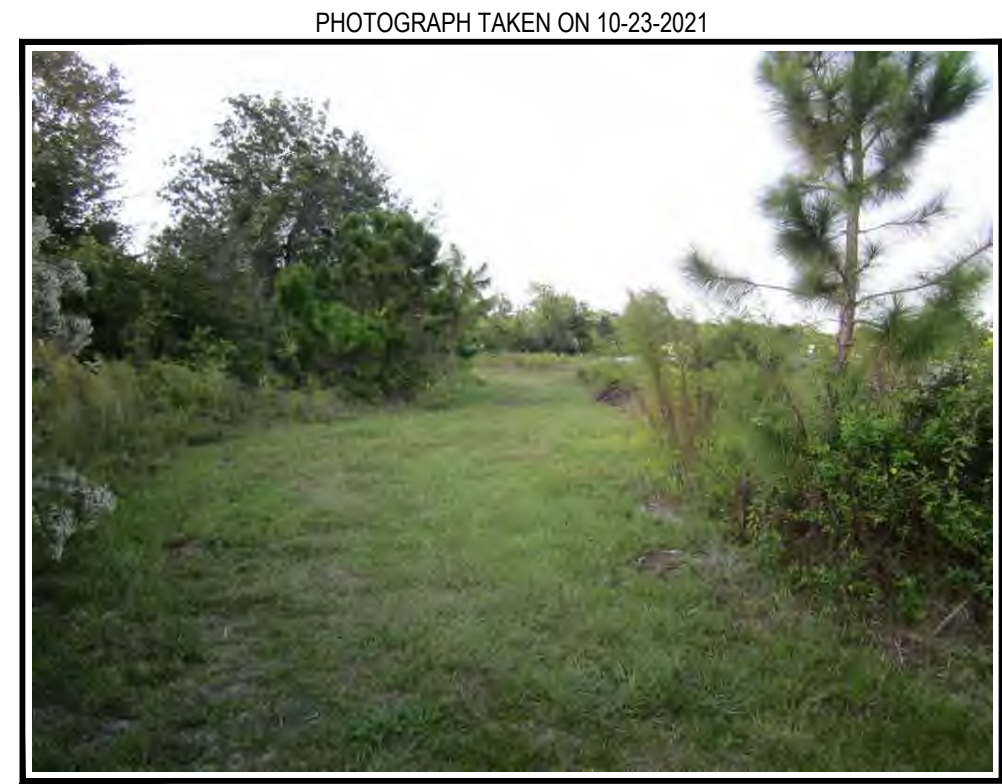
VIEW OF THE RE-ALIGNMENT CORRIDOR LOOKING NORTH FROM 3216 / 3220 OXBOW COURT
