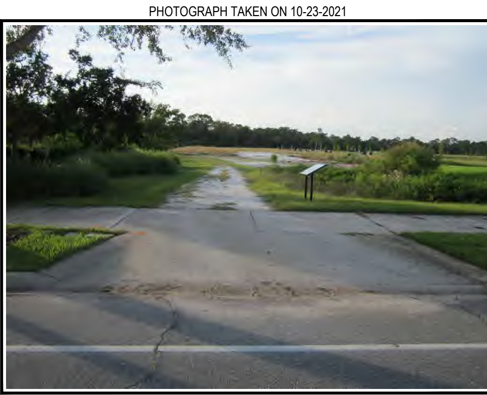
EXISTING CONCRETE DRIVEWAY AT FIVE OAKS DRIVE
