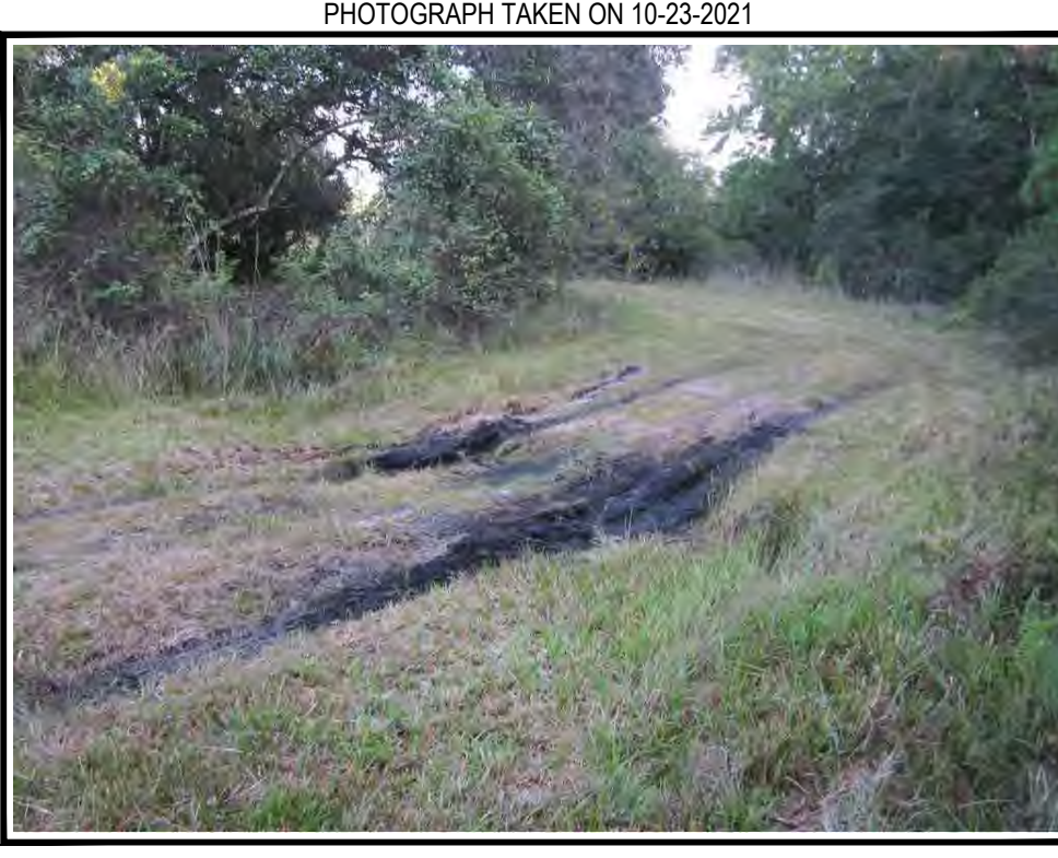
EXISTING LOW POINT AND OVERFLOW FOR CONSERVATION TRACT 4 LOOKING SOUTHEAST
