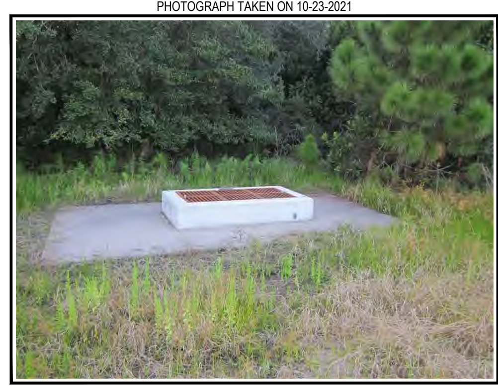
EXISTING OVERFLOW STRUCTURE AND CONCRETE APRON
