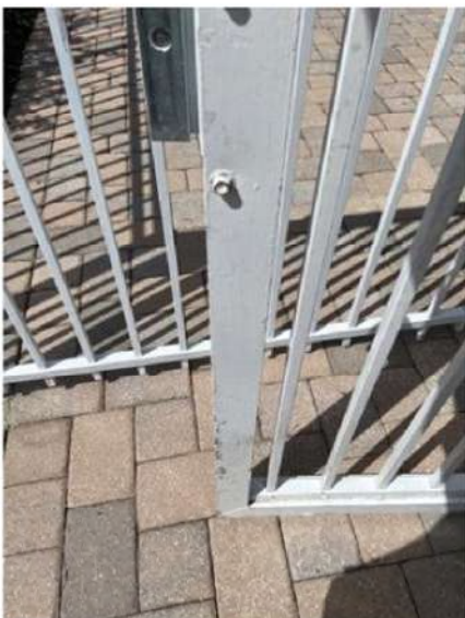
Observation 25 Sand and paint gate swim club
