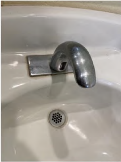
Observation 17 Clean and polish faucets
