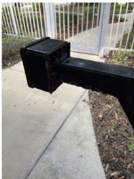
Observation 32 Scrape paint off and sand and paint at Ashley
