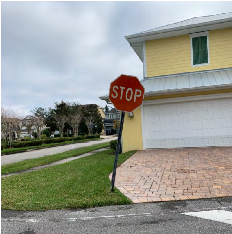
Item 31 Assigned To ? Stop sign post needs straighten or replaced behind 7125 Indiagrass
