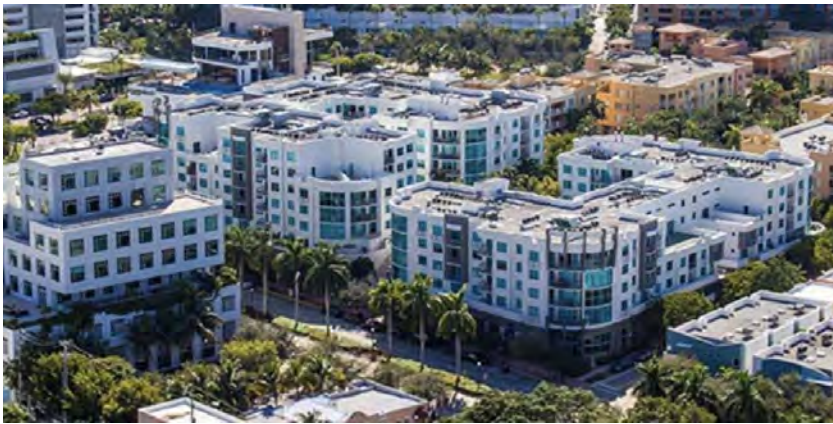
Portofino Towers 1-5 & Master Association, Pensacola Beach
