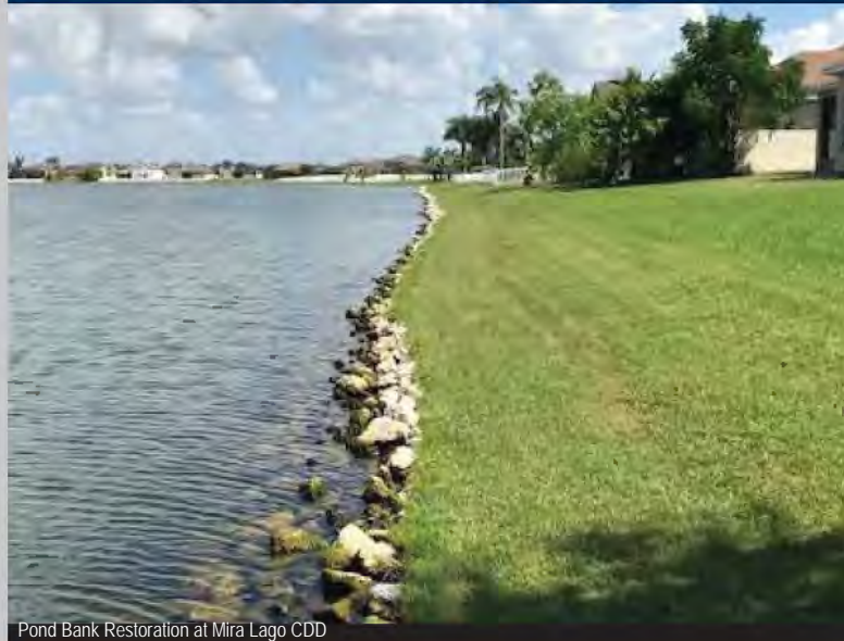
Pond Bank Restoration at Mira Lago CDD
