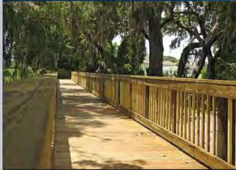
Pedestrian Boardwalk at Oak Creek CDD
