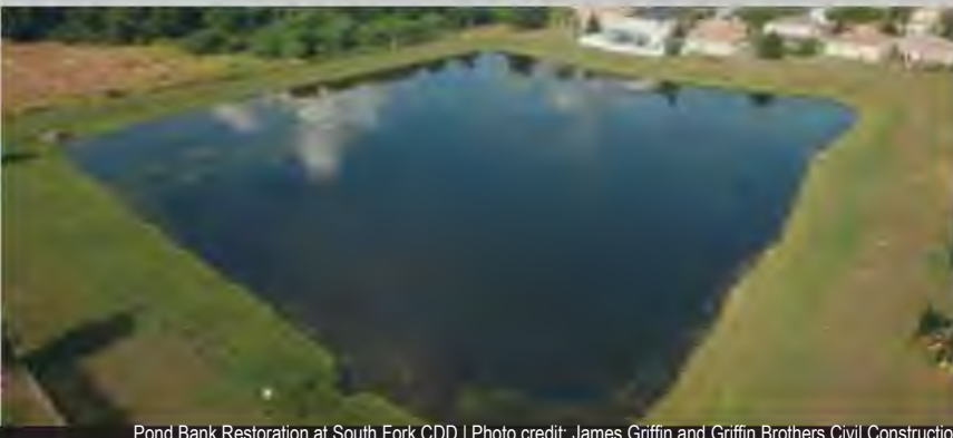
Pond Bank Restoration at South Fork CDD | Photo credit: James Griffin and Griffin Brothers Civil Construction
