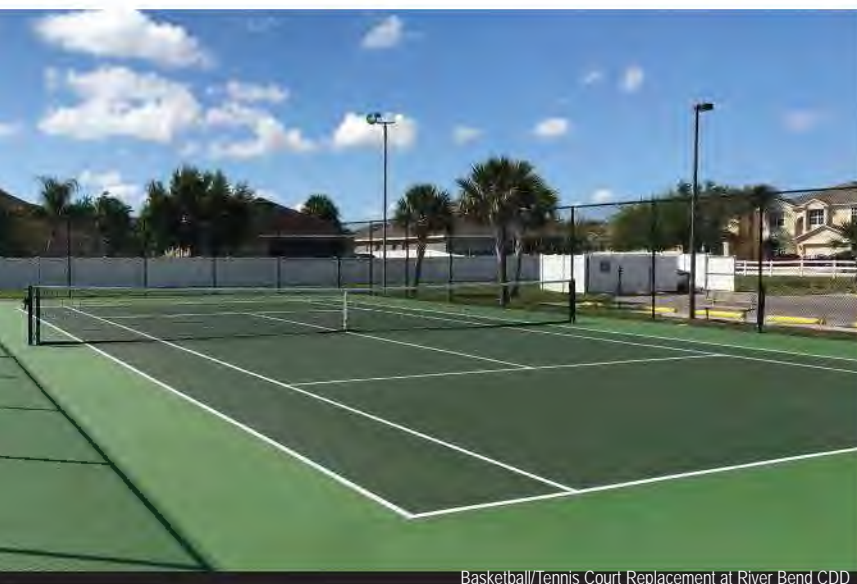
Basketball/Tennis Court Replacement at River Bend CDD
