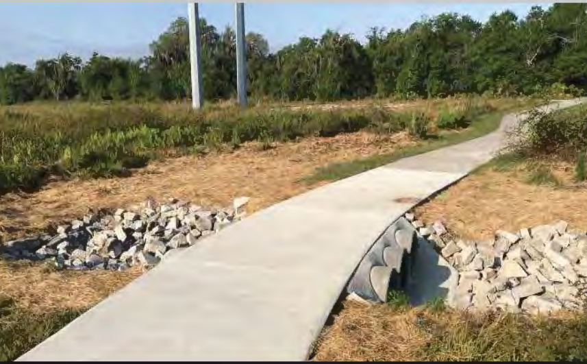
Sidewalk Repairs at Fishhawk Ranch CDD
